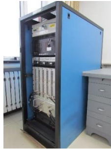
(Below) 20 kW EMDR showing transmitter in lower section
