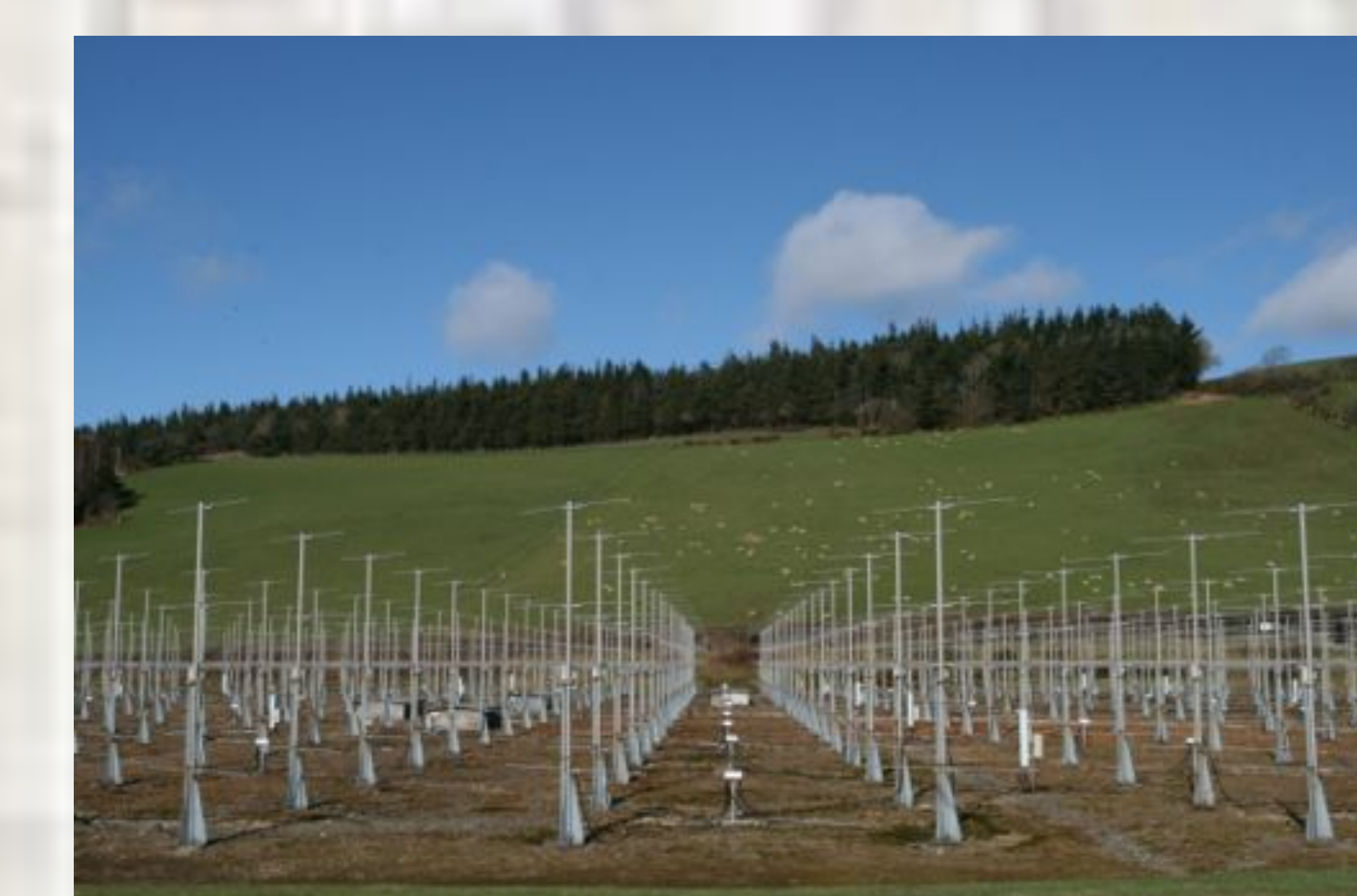
Fig14. View of the antenna array after the installation
