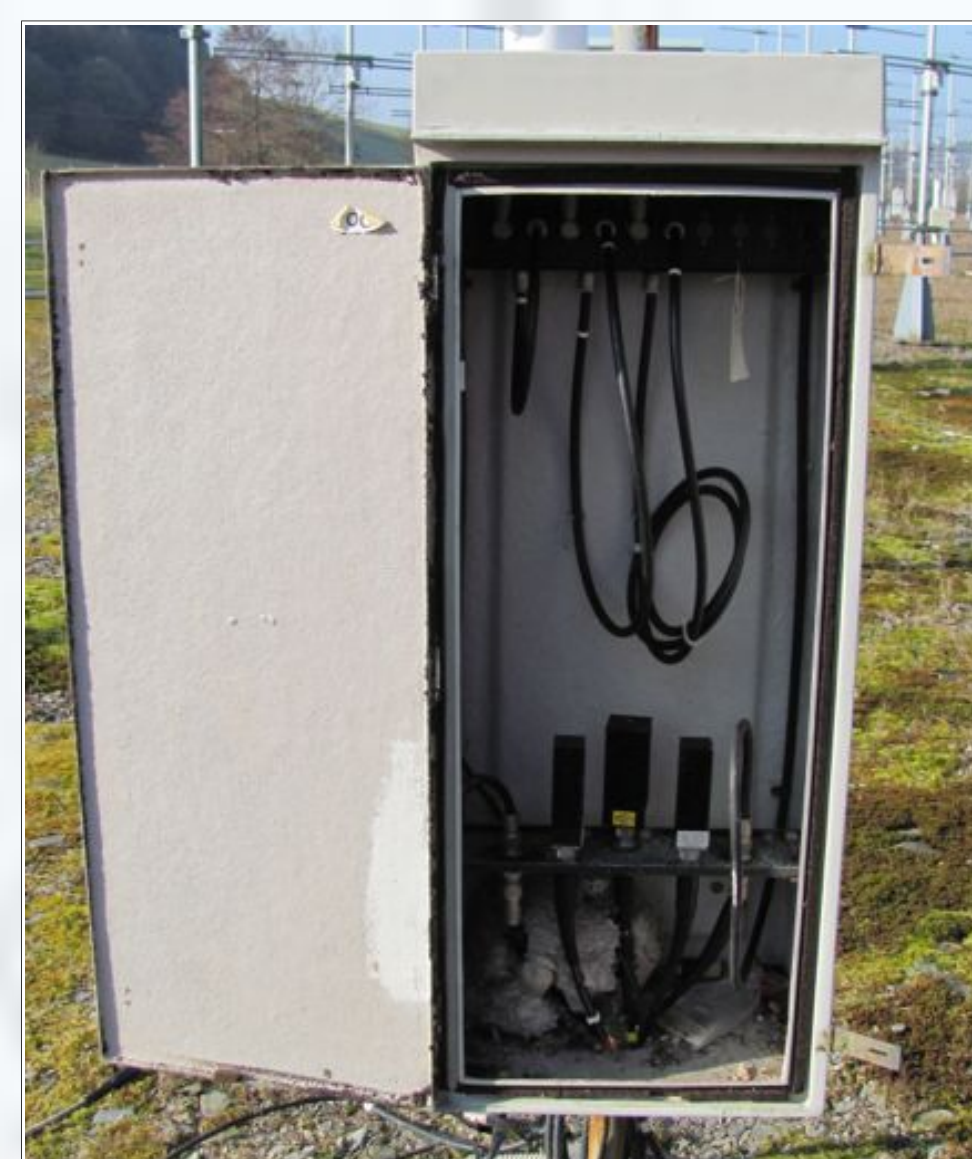
Fig3. Side view of an old Phase Shifter unit showing the associated 4-Way Splitter.
