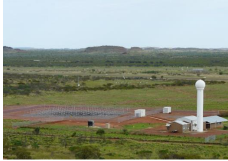
(Above) The Tennant Creek STP, alongside the weather watch radar. The STP system is an 80-kW peak power, 144 Yagi antenna array, single receive channel radar, which operates in DBS mode. The antenna array covers an area of 40m x 40m. Data are provided by a 30-min BUFR data stream for weather forecasting and numerical weather model assimilation. Higher resolution data are available for basic research purposes
